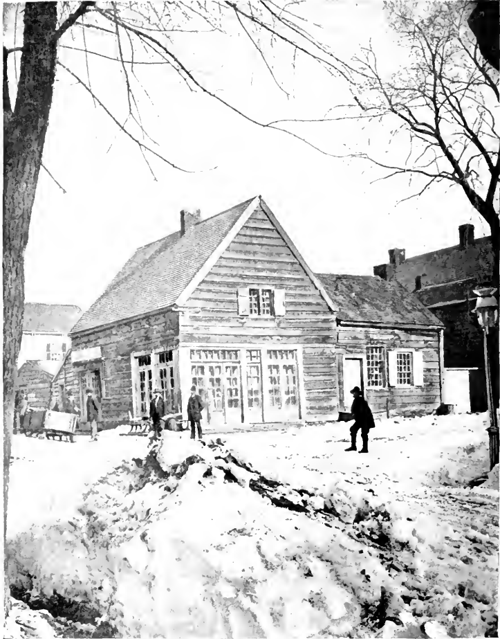
Corner of Washington Avenue and State Street.
